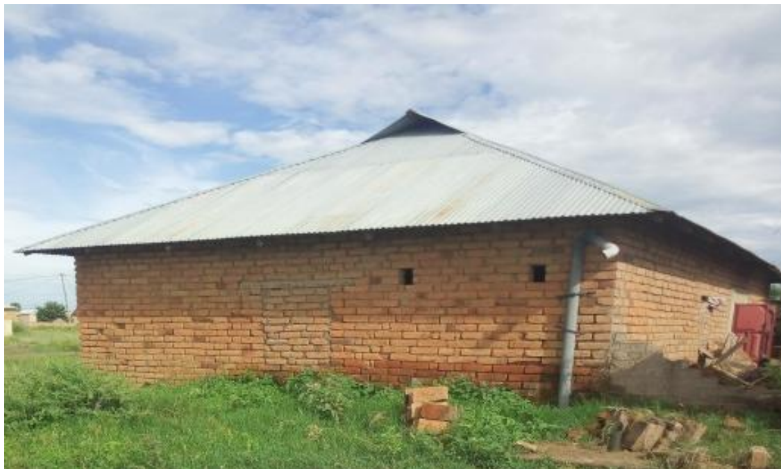
Photo 2: The current view of Mrs Mligo's new house from a distance. Credit: Didas Kimaro
